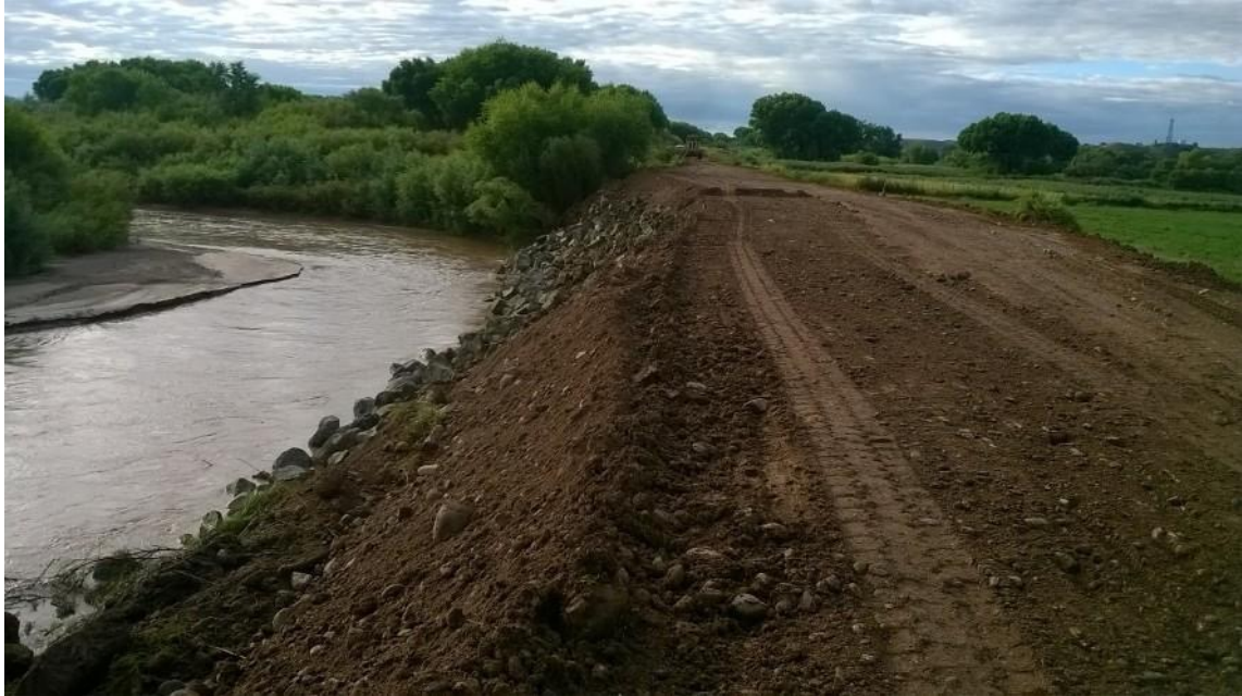
Figure 3: Current dikes in place. [8]
